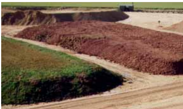
Clearly defined stockpiling of different soil materials
