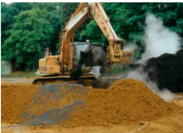
Blending organic matter with mineral material
