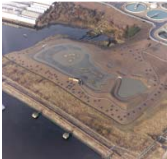
(Northumbrian Water) Using spoil waste to create wetland as part of a £70m improvement to Howden Sewage Treatment Works avoided the need for some 16,000 heavy lorry journeys through the local community and saved £1.152m.
