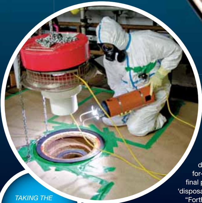
**TAKING THE TUBE:** The Avexis is lowered through a six-inch aperture into the silo liquor below.
