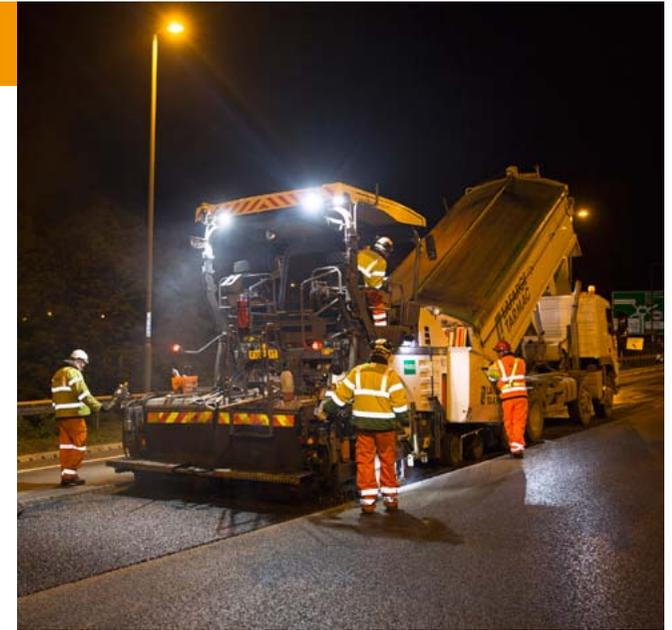
Running through an urban area, the single carriageway road has numerous side roads and mini roundabouts and the work had to be done under off peak daytime lane closures – although access had to be provided at all times for live traffic. The laying of surfacing, 50mm thick following the planing out of a similar depth of existing material, took place over five days. Daily productivity was affected by the laying logistics, not the material Lumley says.
