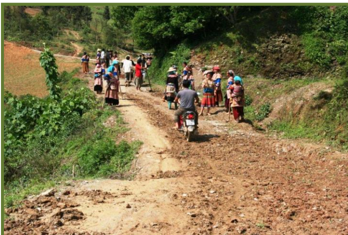
Ethnic minority women engaged in maintenance work on rural roads under the Rural Transport Programme (RT3) in Lao Cai province. RT3 will help improve access to 3,000 communes and lift 320,000 people out of poverty (Source: Phan Manh Tuan, RT3 Consultant)
