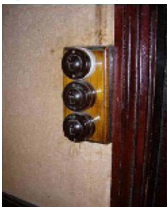
**Fire hazard – old wiring:** increases the risk of a fire starting (and electrocution).
