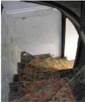
**Risk from fall on the stairs:** steep, narrow winding with no handrail.
