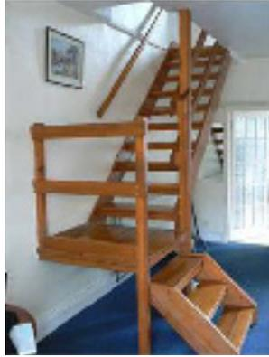
**Risk of falls between levels:** large gaps in balustrade and insufficient area of platform part way up.
