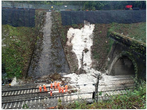
Figure 5: View of landslip and debris on track. The adjacent masonry structure is a face wall (refer to paragraph 90).
