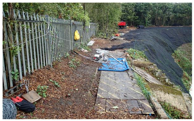
Figure 13: Concrete raft above face wall. Scaffolding boards had been placed inside the raft to remove a tripping hazard during the slope protection works.
