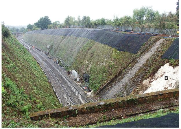
*Figure 7: View of slow lines cutting from above tunnel portal, looking north-west towards Gypsy Lane bridge on 16 September 2016. The partly completed slope protection works are visible. The landslip is marked 'B'.*
