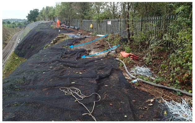
Figure 9: Crest of cutting above landslip showing erosion matting displaced by surface water flow
