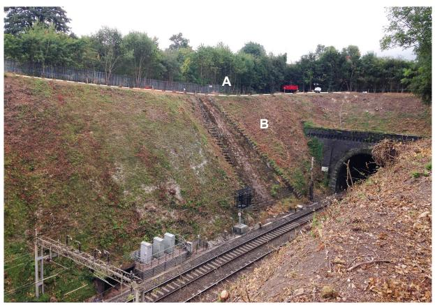
Figure 6: Photograph of cutting taken in July 2016 following vegetation clearance looking east (courtesy of Network Rail). The white dashed line indicates the profile of the cutting crest with the low point marked 'A'. The location of the future landslip is marked 'B'.
