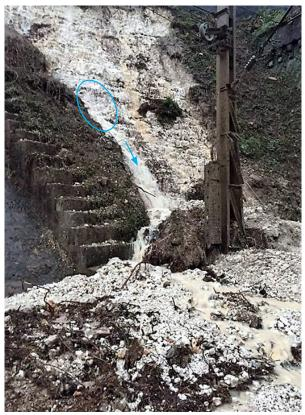
Figure 10: Image showing water emanating from part-way down the cutting slope (courtesy of Network Rail)
