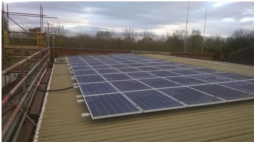
This project undertaken in 2016 involved the installation of photo voltaic cells to the main garage roof providing 15KW of power generation connected to the incoming electricity supply via metering located in the LV Switch Room. . It was anticipated that the saving to the Trust will be £3,385.00 per annum on this site (based on current unit/hour rates).
