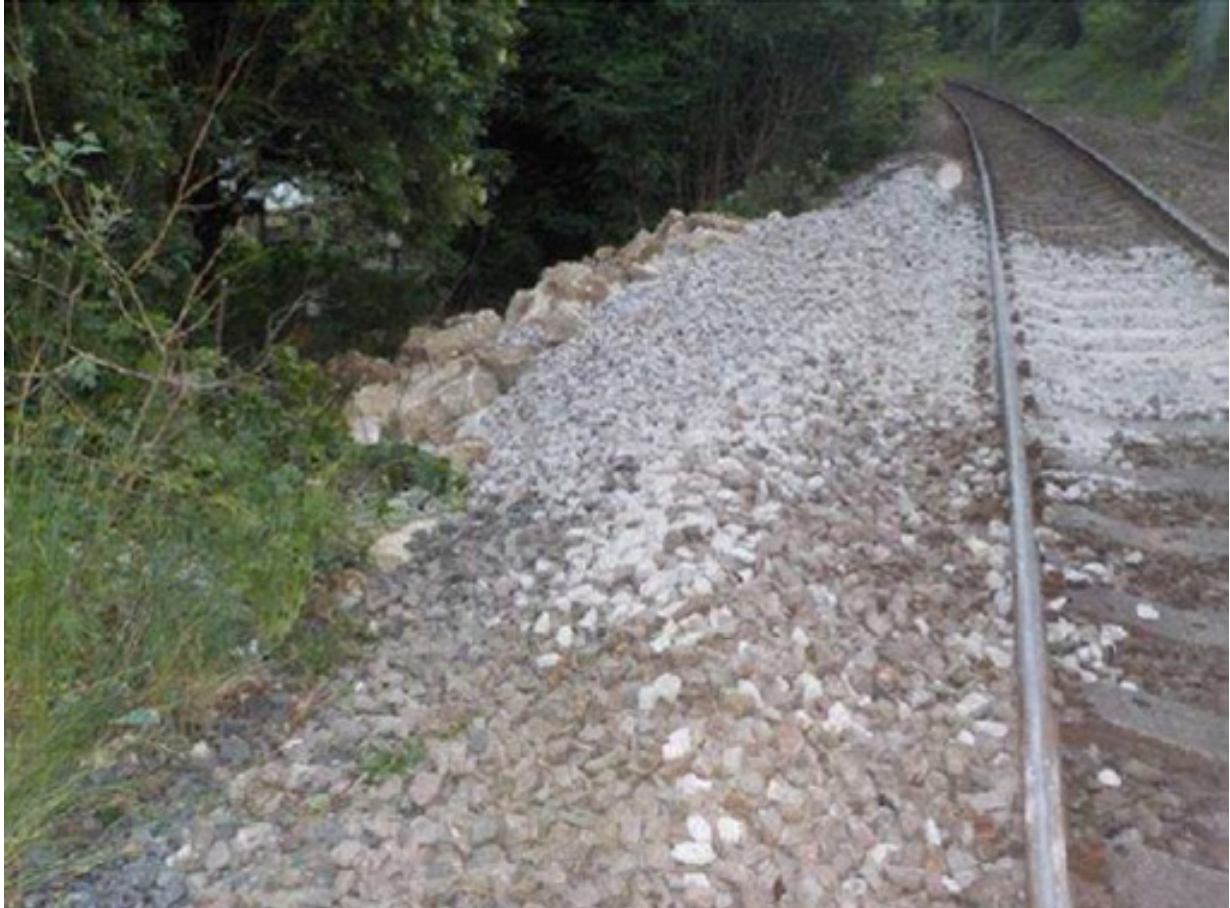
Figure 9: The rebuilt embankment following its repair
