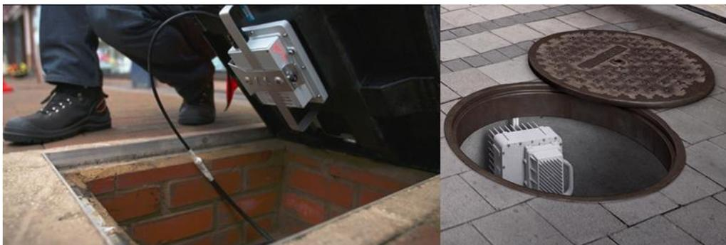
Figure 31: Pavement deployment of small cells. Source: 3G4G Small Cells Blog<sup>68</sup>
