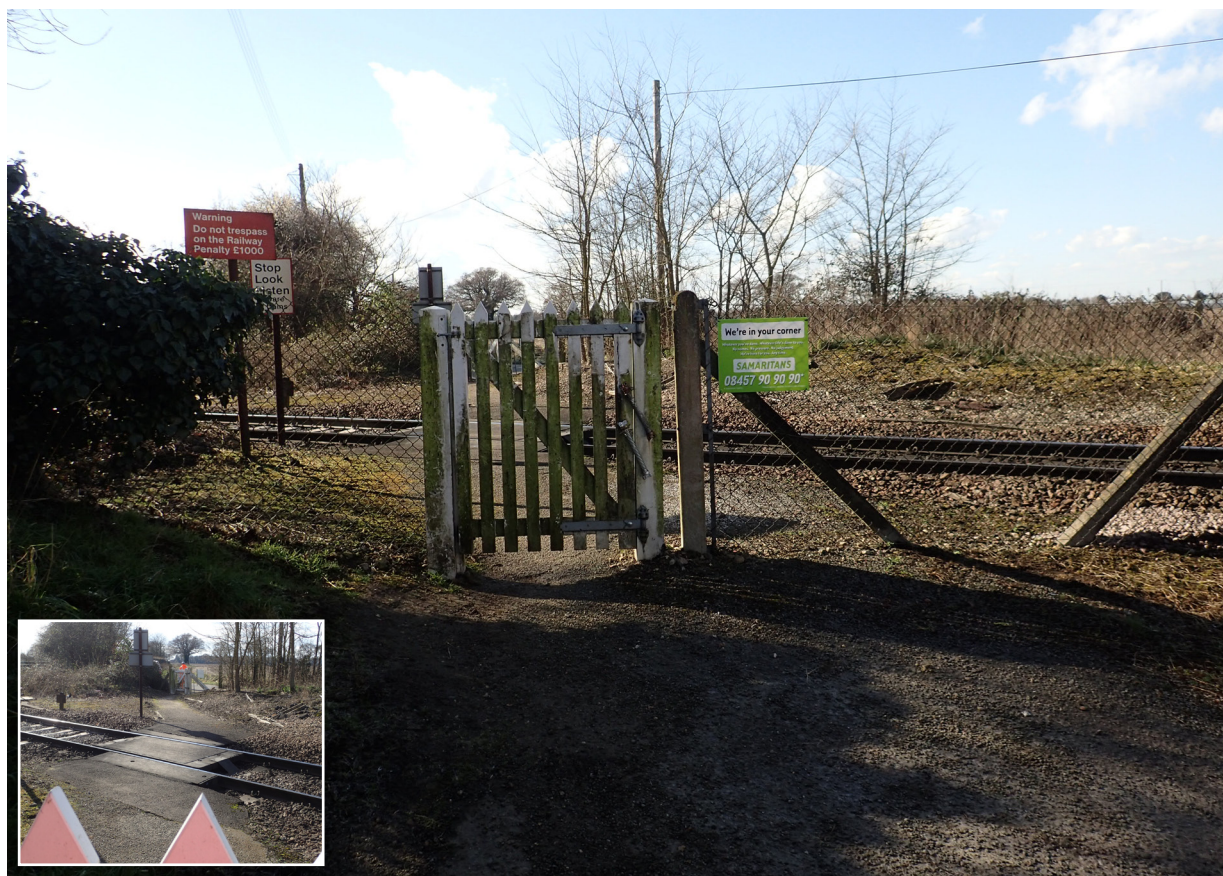
Figure 6: Key features of Grimston Lane footpath crossing when approaching from the east
