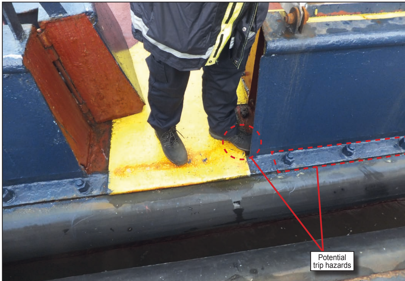
Figure 6: Bulwark structure, fendering and securing bolts
