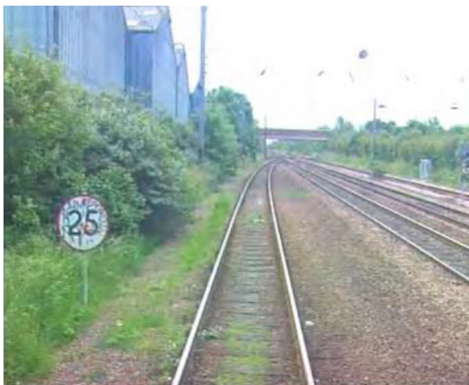
Figure 11: Full-size permissible speed indicator at Fletton Junction in 2002 (image courtesy of Network Rail)
