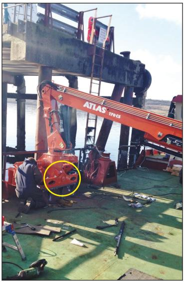
Figure 17: Crane installation showing inboard box section (circled)
