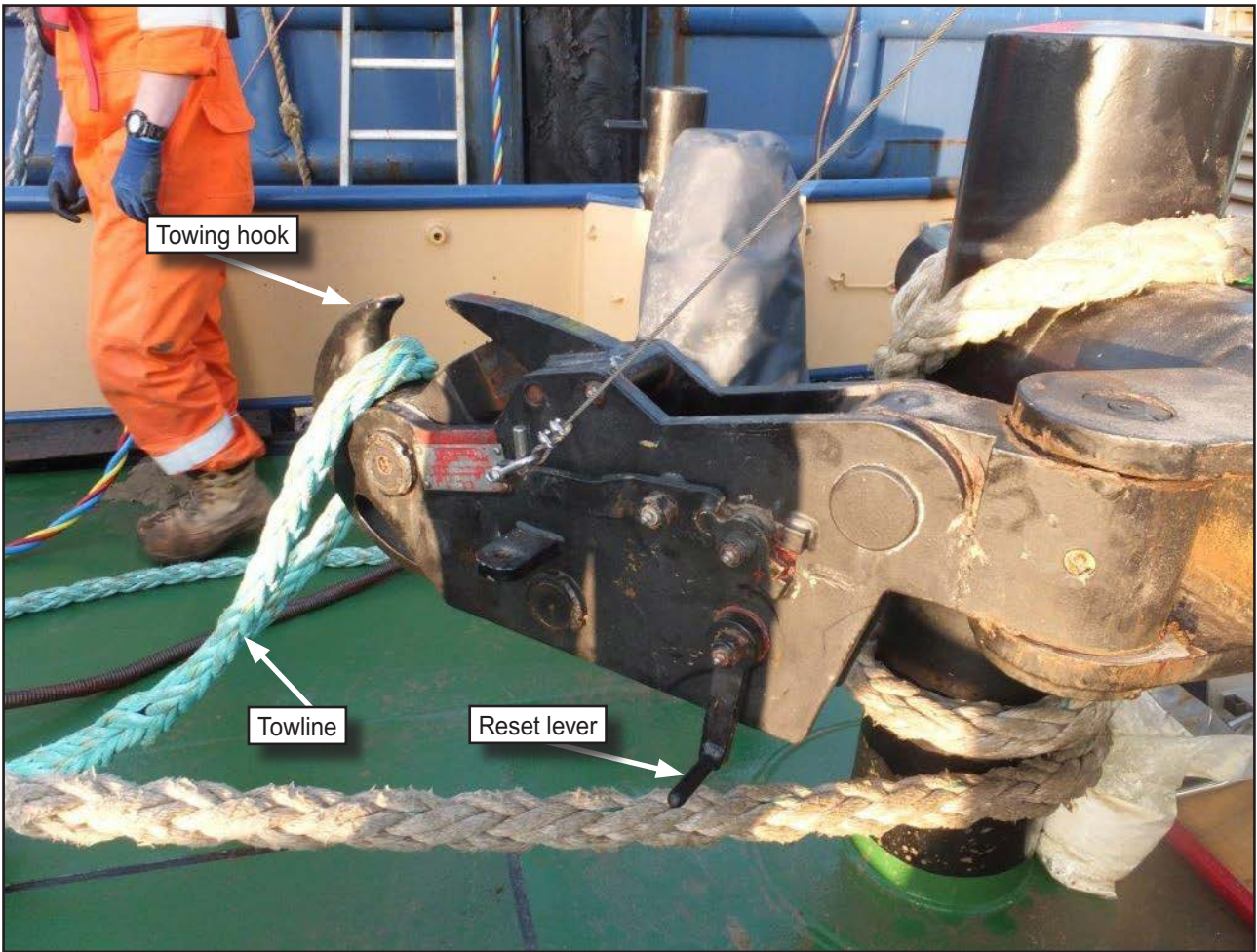
Figure 7: Towing hook (as found following salvage)
