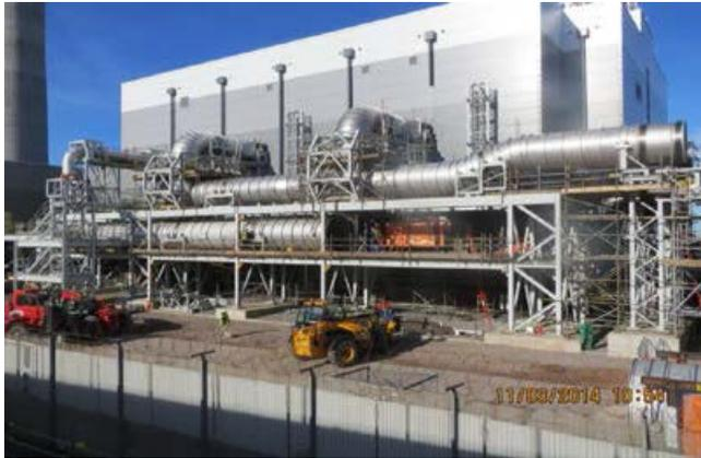
This project is to divert the existing vent streams from the processing plants at Sellafield away from the Windscale Pile Chimney to a new discharge facility located outside the Separation Area. This will allow demolition of Windscale Pile Chimney stack to be completed. The new discharge facility will comply with modern discharge authorisations.
