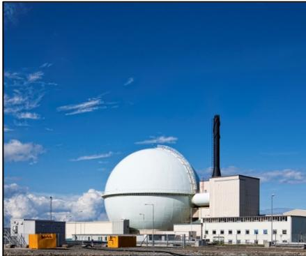
Dounreay was established as a research site in the mid-1950s with fuel production and processing facilities. There were three reactors, the last of which ceased operation in 1994.
