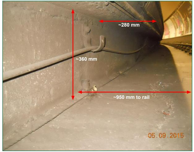
Figure 20: Clapham South platform recess
