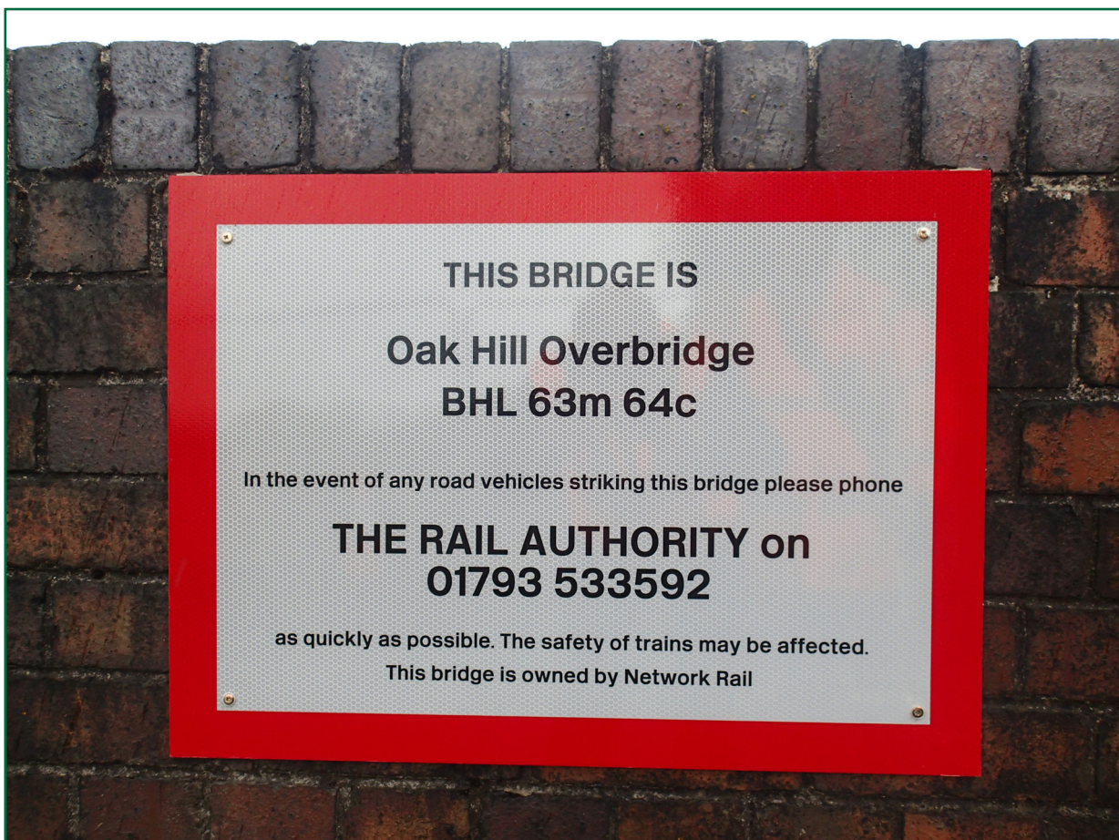
Figure 11: Bridge identification plate fitted to Oak Hill Road overline bridge after the accident
