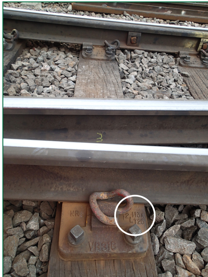
Figure 7: Two-levelled baseplate with marking (circled) to show it is 25 mm thicker than the standard baseplate
