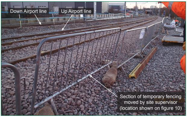
Figure 12: Section of temporary fencing moved to gain access to railway
