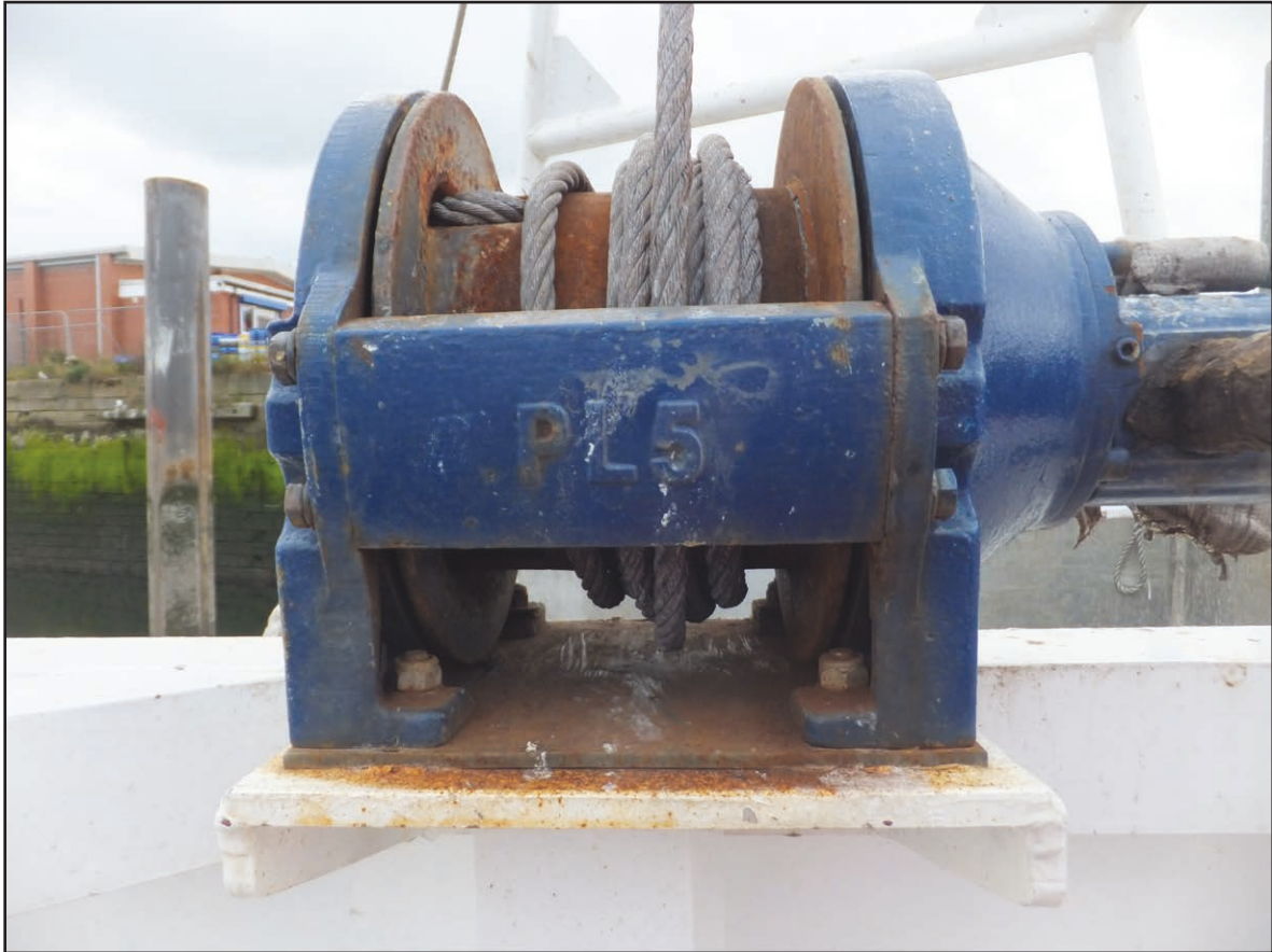
Figure 4: Gilson winch showing build up of wire
