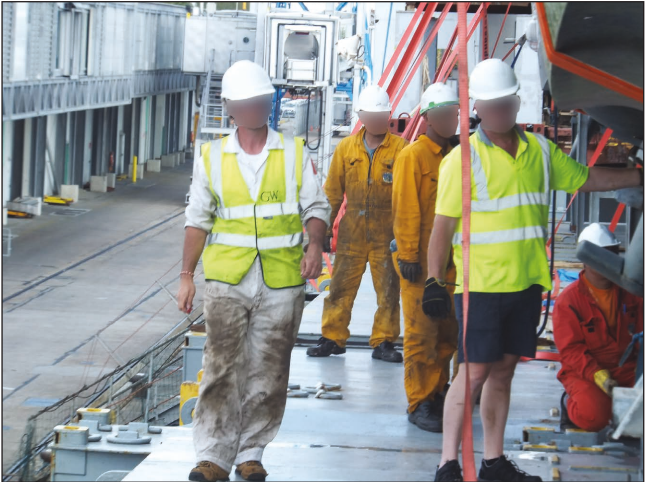
Figure 10: People walking and working close to the exposed edges of the hatch covers
