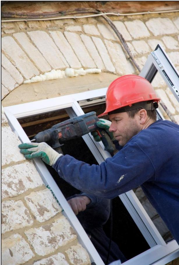
Picture 6 - A local installer installing double glazing windows in a PAYS household
