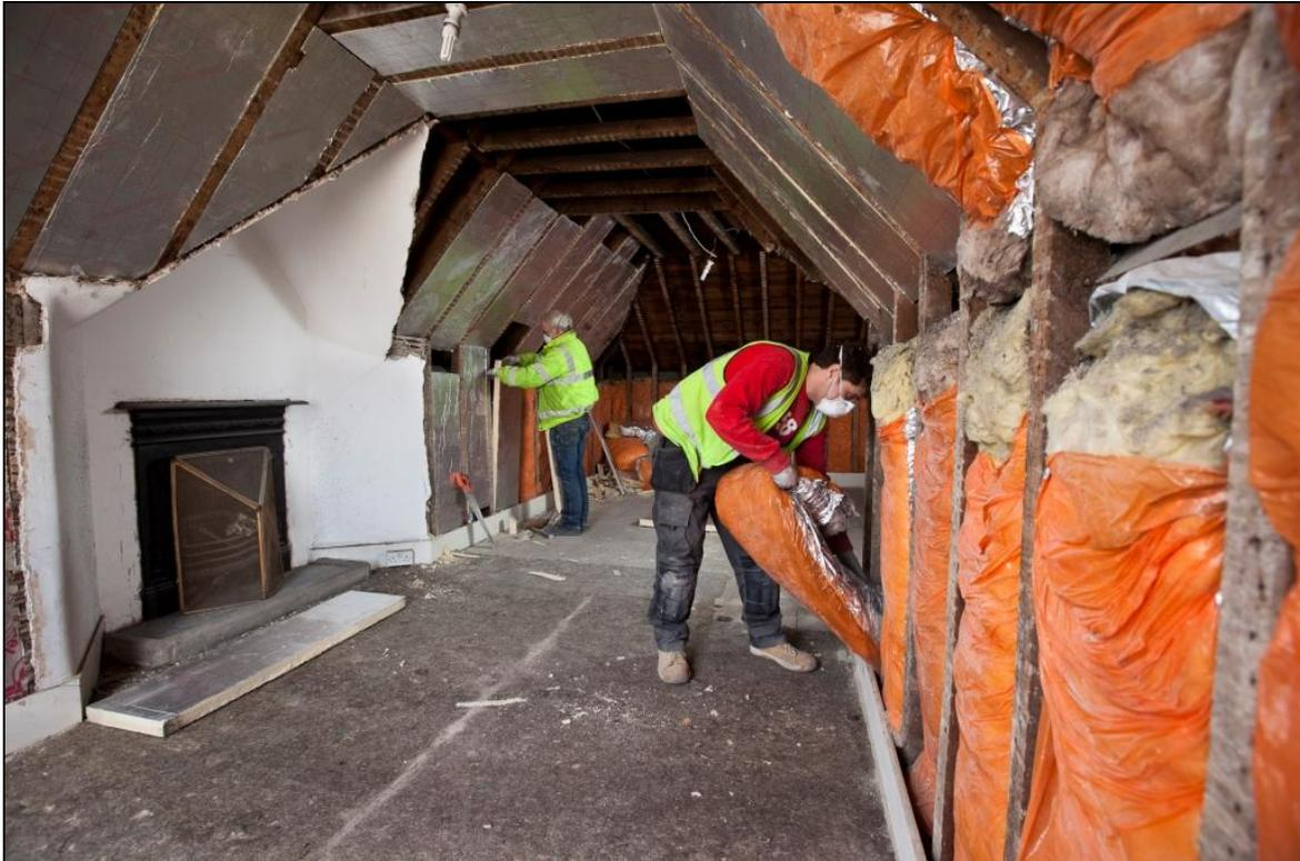
Picture 1 - Sloping ceiling and loft insulation installed in a PAYS household
