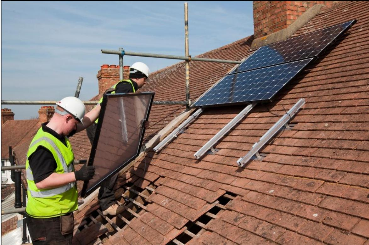
Picture 2 - Installers laying Solar PV Panels in a PAYS household
