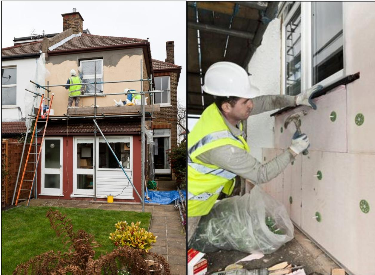
Picture 4 & 5 - External solid wall insulation installed in a PAYS household
