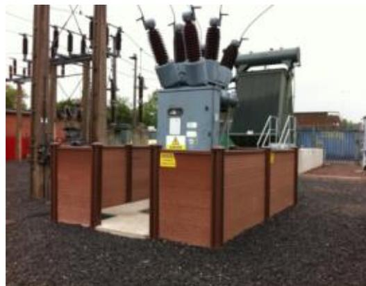
Since 2010 we have been designing for flood risk at all our new substations, including smaller distribution substations. The usual mitigation for a new site is to place equipment on raised plinths to ensure it remains above the predicted level of any flooding.
