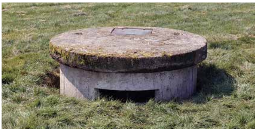
The turret of a Pickett-Hamilton Fort, a type of retractable pillbox, restored at RAF Honington © Honington Herald
