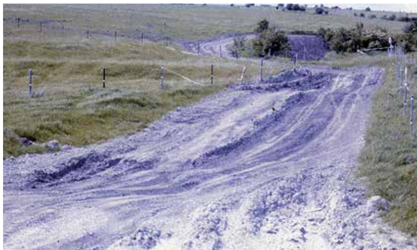
Surface damage caused by vehicle movement in wet conditions. © Wiltshire Council
