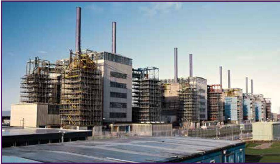
Since the project began eight years ago, 3,300 tonnes of asbestos have been removed from the turbine hall, four reactor buildings and 16 heat exchangers. More than one million bags of asbestos waste (equivalent to filling four Olympic-sized swimming pools) were despatched to licensed landfill sites.
