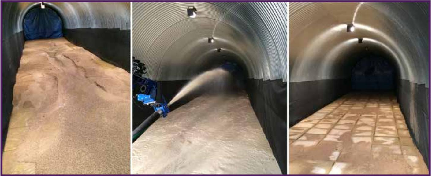
A remotely operated water cannon will wash out sludge from a tunnel section of Dounreay's shaft and silo complex, following a series of trials to test the novel approach.
