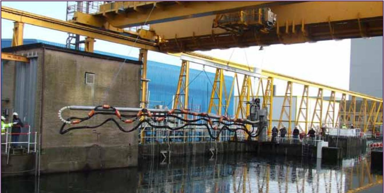
The Sludge Retrieval Hood in operation at the open air pond
