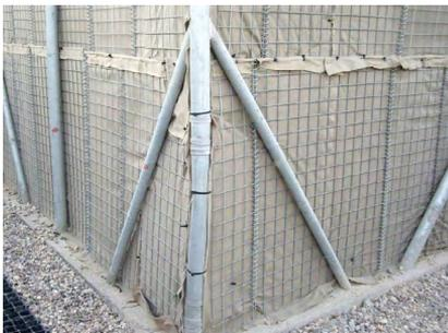
a. Ensuring that the bases of all fences are embedded in a concrete ring beam that is sunk at least one foot into the ground. Engineer advice will be needed to take into account local conditions. The image opposite shows a welded mesh fence, fixed to the inside of posts and sunk into a concrete ring beam.
