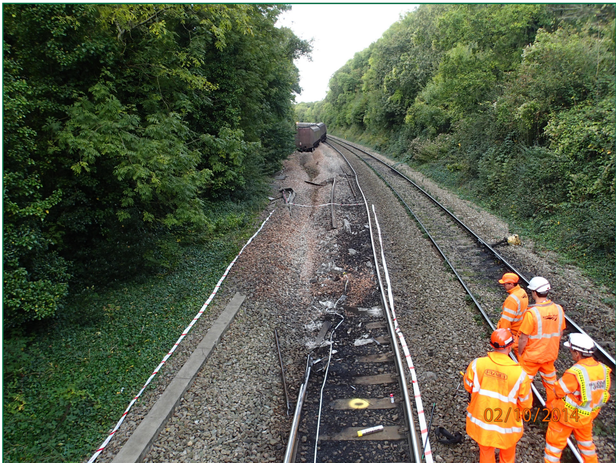
Figure 2: Overview of derailment site
