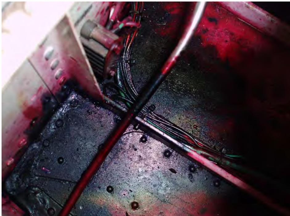
Cover photo shows zonal contamination due to fluid leakage surrounding electrical terminal blocks.
