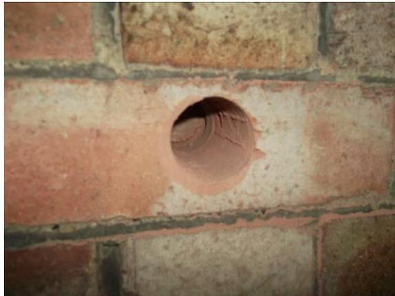
Figure 5: An area where a core sample was taken. The gap between the inner and outer stretchers is just discernible as a shadow at the back of the bore hole.
