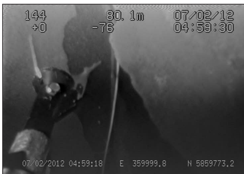
Figure 2: ROV image of the structural failure amidships
