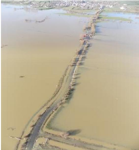
The County Council scheme is being carried out in two phases: This autumn a breach approximately 12m wide has been cut through the road to allow flood water to pass under it. A temporary bridge has been installed to allow traffic to use the road which has been resurfaced and raised as appropriate. In spring 2015 the breach will be replaced with a set of two culverts. Two more culverts will then be placed further along, and the road reinstated.
