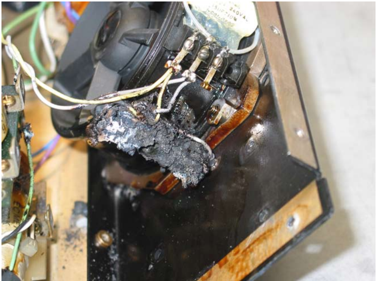
Figure 1 Burnt out capacitor
