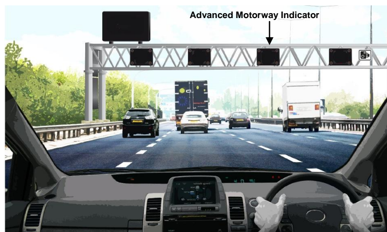
Figure 4A: Illustrative M1 junction 19 to 16 smart motorway all lane running scheme section operating in normal motorway conditions with blank advanced motorway indicators and blank gantry mounted variable message sign
