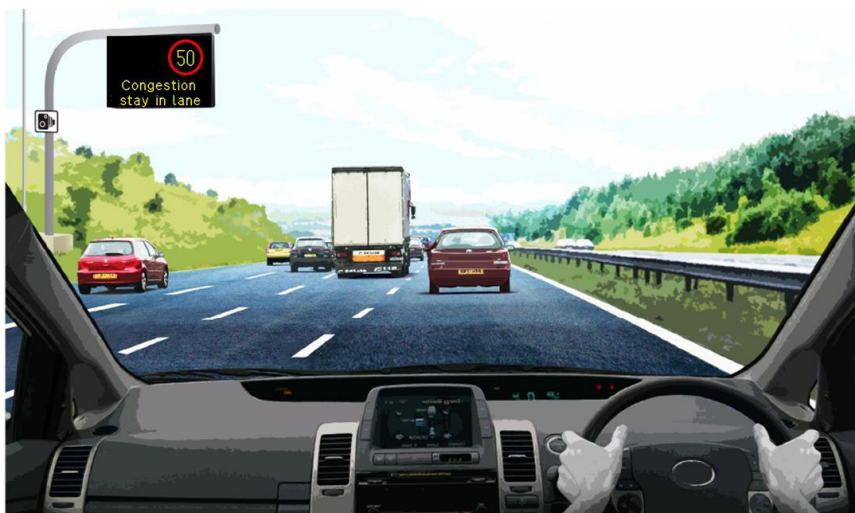
Figure 4D: Illustrative M1 junction 19 to 16 smart motorway all lane running scheme section operating with variable mandatory speed limits and information for road users.
