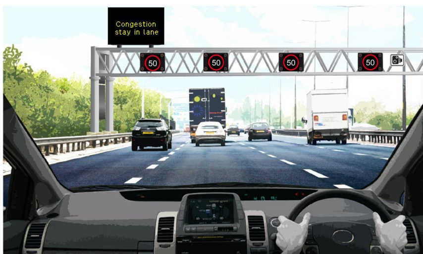
Figure 4C: Illustrative M1 junction 19 to 16 smart motorway all lane running scheme section operating with variable mandatory speed limits
