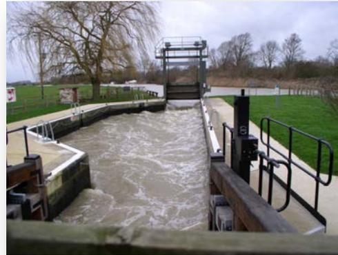
The photograph above shows how a lock may be used to discharge flood water on the River Great Ouse when Strong Stream Advice has been issued.
