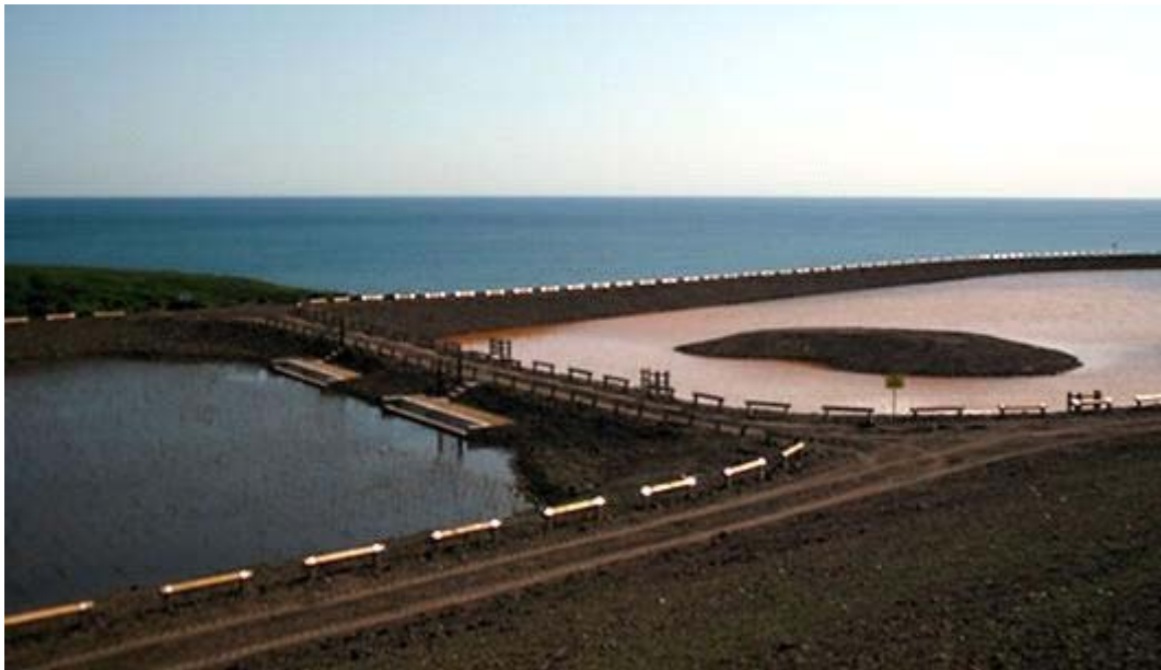
The Coal Authority Photograph – Pumped Passive Mine Water Treatment Scheme Horden, Durham,
