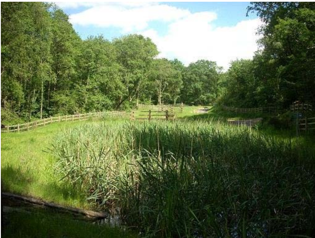
The Coal Authority Photograph - Passive Mine Water Treatment Scheme Tan-Y-Garn, adjacent to the River Cathan, north east of Garnswilt, near Ammanford, Carmarthenshire
