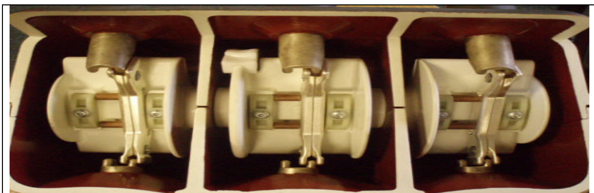
Figure 2: 200A/630A Disconnecter Contacts
