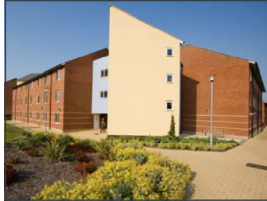
Single Living Accommodation at Tidworth
