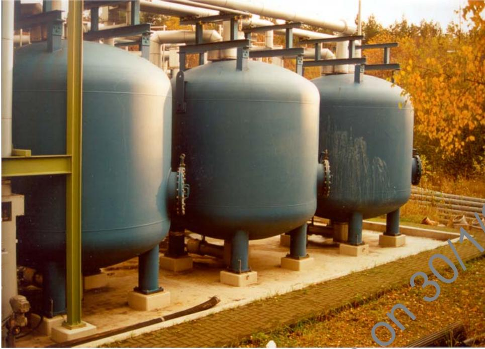
**Plate 2.9:** Typical external sequential GAC tank installation for polishing of biologically-pre-treated landfill leachate
