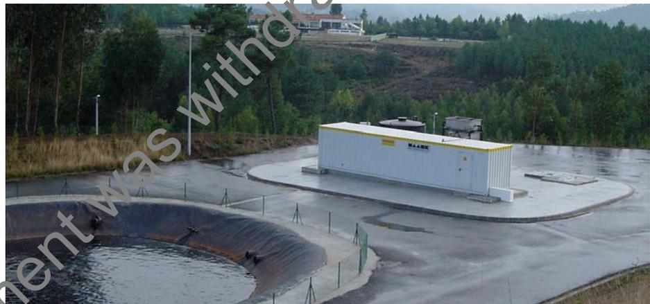
**Plate 2.5:** Typical configuration of a 2-stage RO plant with aerated leachate lagoon, direct permeate discharge and concentrate re-infiltration (120 m<sup>3</sup>/d, Rebat landfill, district of Amarante, Portugal, commissioned 2001) (see Loeblich 2005)
