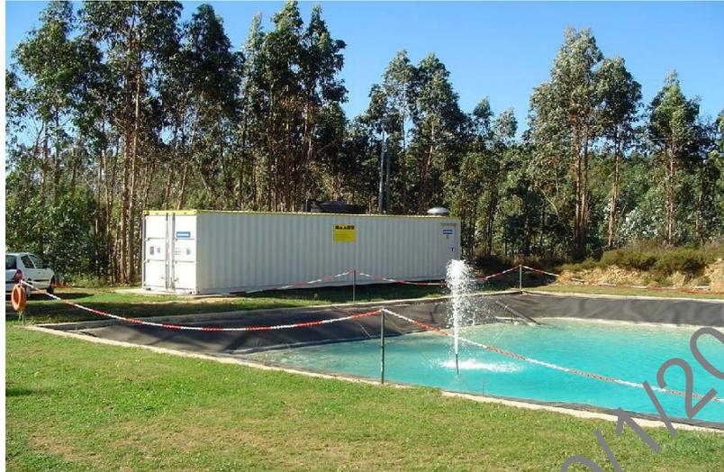
**Plate 2.4:** Typical configuration of a 2-stage RO plant with permeate lagoon (140 m<sup>3</sup>/d, Tondela landfill, district of Tondela, Portugal, commissioned 2004) (see Loeblich 2005)
