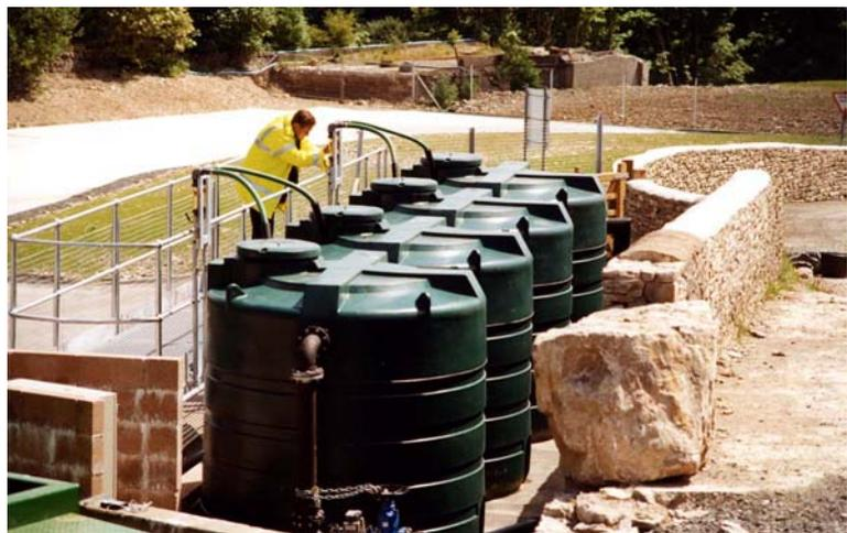
**Plate 2.1:** Typical methane stripping plant, treating up to 300 m<sup>3</sup>/d of landfill leachate, at Kendal Fell Landfill, Cumbria, 2002
