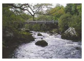
D3e Minor bridge – pipelines crossing rivers, if lacking central piers, are recorded as minor bridges. See also Na. Note exposed boulders and broken standing waves.
