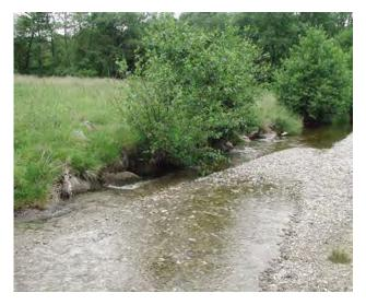
I6a Reinforced bank – toe only; reinforcement is with large boulders (rip-rap). See also E1Ja,b, E1Ka, E1Oa.
