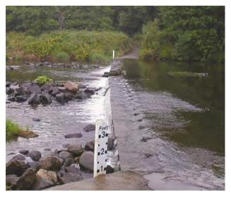
D5a Major ford – both the bed and banks are made of artificial material, and there is obvious ponding of water upstream.
