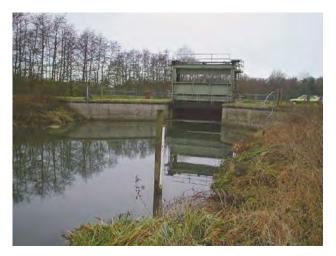
D1b Major weir/sluice – sluice; settings can be changed to influence water levels upstream. Water is impounded upstream.
