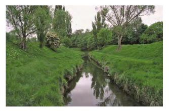
E2Ca Artificial Berm – formed by excavating bank material (here on both sides) to form a two-stage channel. Both the flat base of the berm, and the face of the top of the bank, constitute 'bankface'. See also E1Hb, F18b.
