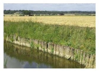
E1Jb Wood piling bank material – vertical poles below resectioned bank and arable (tilled) land-use in background.
