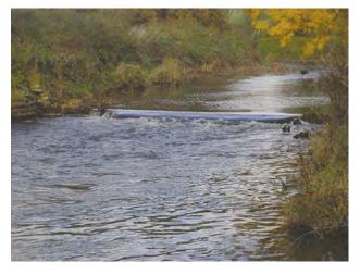
D9a Is water impounded by weir/dam? Photo shows water artificially impounded behind a shallow weir structure. See also D1b,c, D5a.
