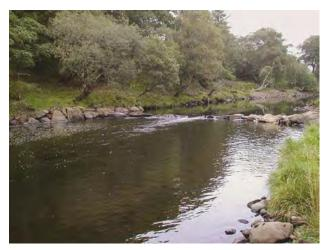
D1e Intermediate weir – boulders are not cemented, and water can leak through the fissures.
