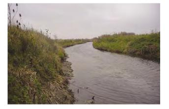
E6b Resectioned channel – typical signs include trapezoidal 45 degree banks and no trees.
