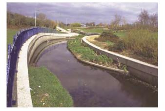
E2Cb Artificial Berm – formed by infilling wide, totally artificial, channel (here on both sides) to form a two-stage channel.
