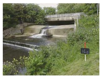
D1d Major weir/sluice – example of a complex weir structure used for measuring flow. Note also an intermediate bridge.
