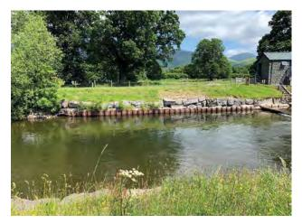
I6b Reinforced bank – toe only; reinforcement is metal sheet piling and rip rap above. Note also bank is resectioned.
