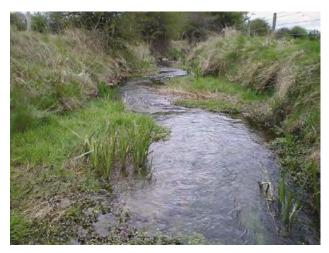
E2Cd Artificial Berm – formed during rehabilitation project by installing shallow shelves (here on both sides) to create a narrower low-flow channel with indistinct berms; note in Section P.
