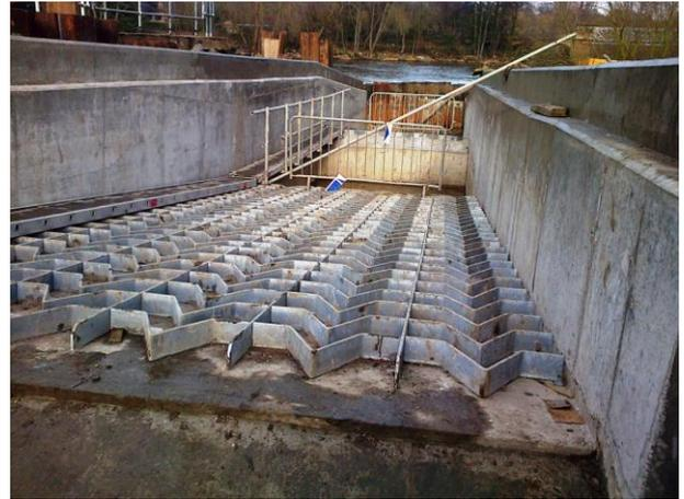
**Construction has finished on the major new fish pass at Sprotbrough, River Don. Once opened, the pass will allow fish access to 8 miles of river upstream of Sprotbrough and at least 3.5 miles of the River Dearne. Coarse fish will be able to reach spawning grounds which have, until now, been inaccessible. The project is a partnership between the Environment Agency, the Canal and Rivers Trust and LaFarge.**
