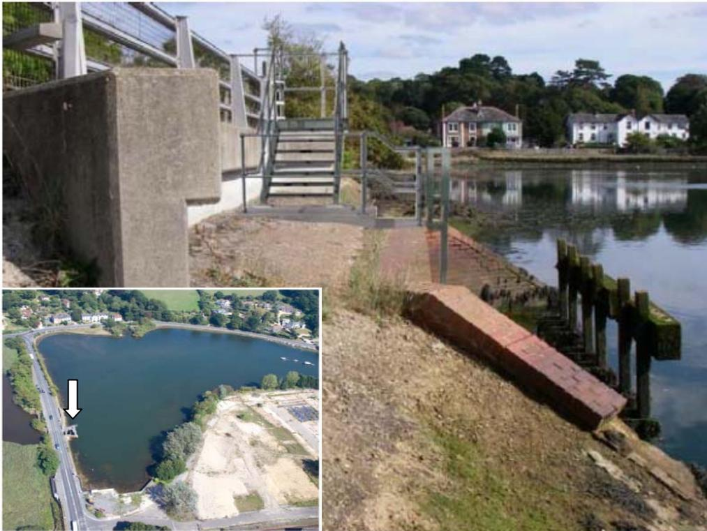
**Figure 3-10 Top-hung tidal flaps at Lymington, furthest one replaced by SRT**
