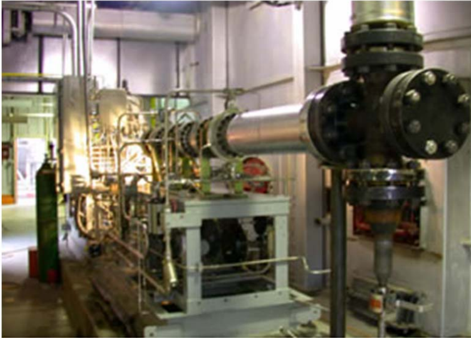
Figure II.3 Original CES burner installation in California; T-piece at end connects to steam turbine
