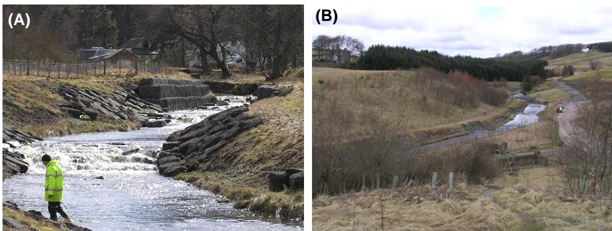
Figure 6. Use of gabions to stabilise banks of the River Nent, Cumbria (A) and re-grading, capping and vegetation of spoil material along the same stretch of river (B)
