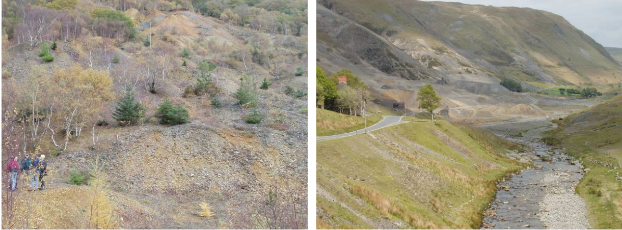
Figure 5. Steeply inclined and unstable mine waste at (A) Cwm Rheidol and (B) Cwm Ystwyth, both in Ceredigion, Wales
