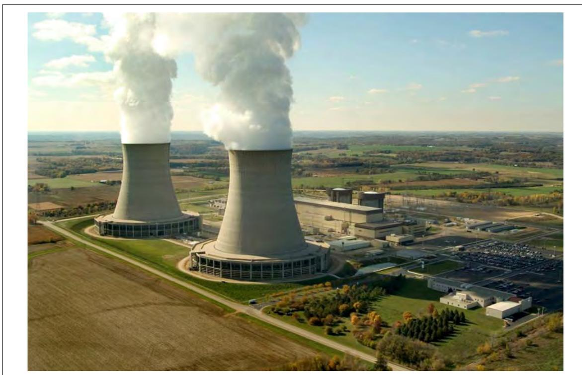
**Figure A3.1 Byron power plant showing the main hyperbolic, wet, natural draft cooling towers fed from the Rock River and the cooling tower 'drift' (by permission of Byron plant)**
