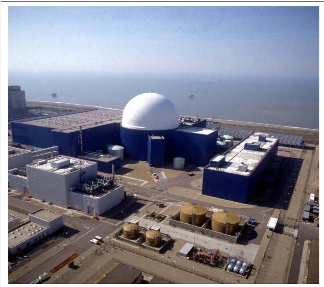
**Figure A2.1 View of Sizewell B PWR showing the North Sea, which is the source of once-through cooling water. A small structure visible offshore is one of the intake structures. Tanks visible are for water, fuel for the diesel generators etc. (by permission of EDF Energy)**
