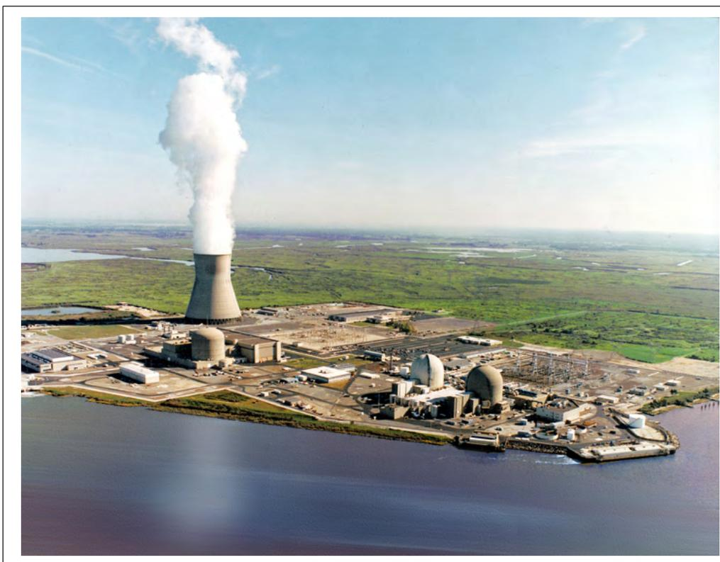
**Figure A3.5 Salem dual reactor site (right) and neighbouring single reactor Hope Creek with cooling tower and associated plume (left) (by permission of Salem Power Plant)**
