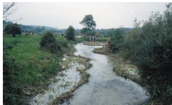
Low-tech rehabilitation on the R. Avon using mattresses to concentrate low flows to the centre of the channel.
