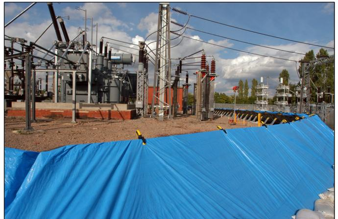
*Temporary demountable flood barrier protecting the National Grid switching station in Walham, Gloucester, the day after the flood inundation in July 2007 (Courtesy of Geodesign Barriers Ltd).*
