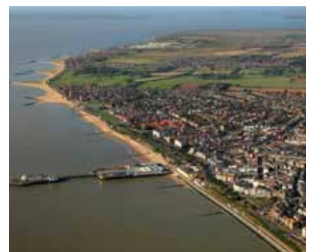
Clacton, and beach control structures at Jaywick (Courtesy of Mike Page)
