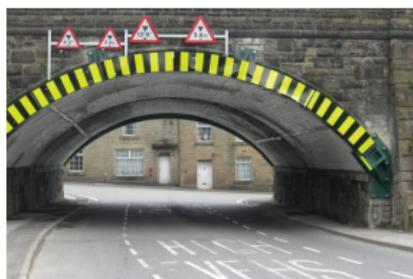
White lines on the road and 'goal posts' on the arch indicating the extent of the signed vehicle height limit
